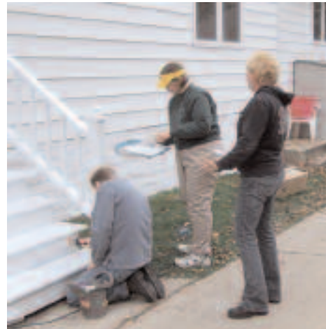
Jackie Olson helping the painting crew.
